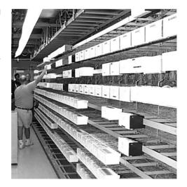
Figure 2-19 Vertical side of MDF, showing protectors
