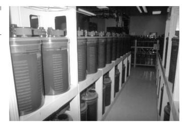
Figure 2-15 Central office battery array
