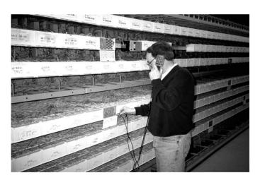
The horizontal side also provides craft/technician access for repair purposes. Each of the white panels shown in the photo flips open to reveal a set of terminals for each wire pair, to which a test set can be connected.
